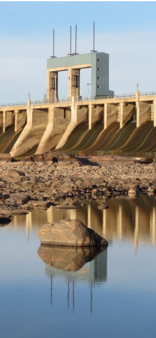
Seven Sisters Falls hydroelectric dam, MB. Photo by James Burns
